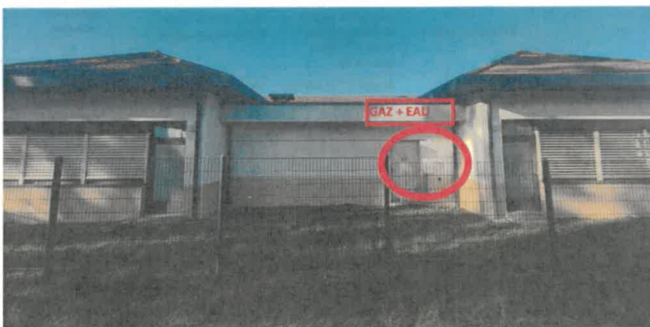
IMAGE 2 (mur SUD extension)
